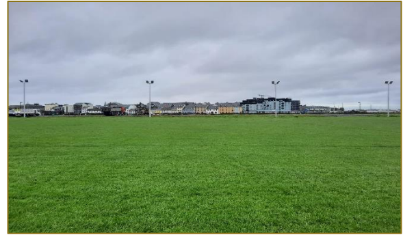
Lighting installation at South Park
