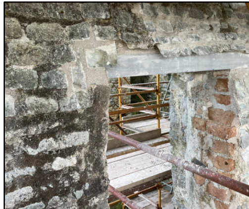
Plates 5 & 6: Lintels replaced and repointing above window openings.
