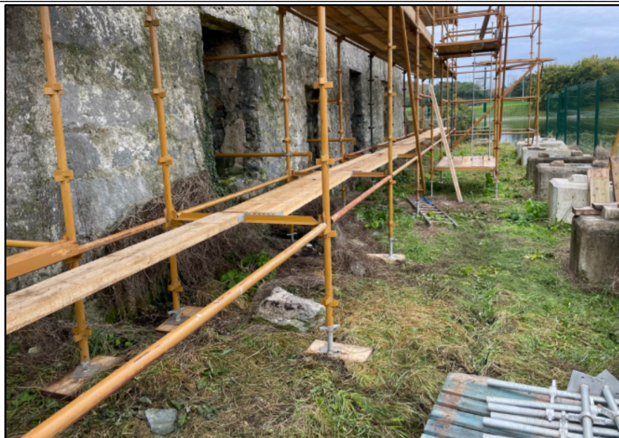
Plate 2: Scaffolding being erected on exterior of W wall of building.
