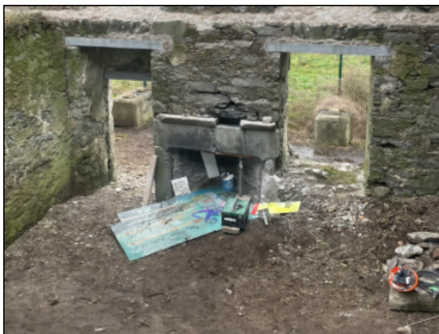
Plate 10: Repair works being undertaken on ground floor fireplace.
