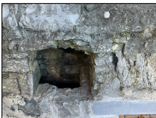
Plates 8 & 9: Repointing of joist hole and work on external finish on upper levels of building.
