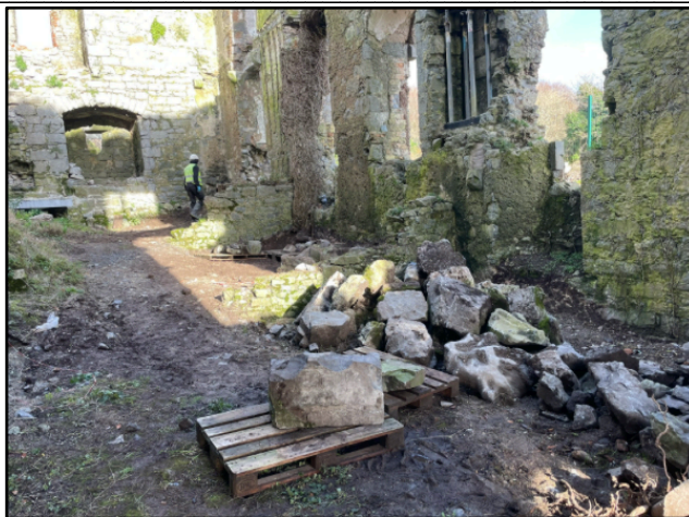
Plate 16: Interior of building from S after sorting stone.
