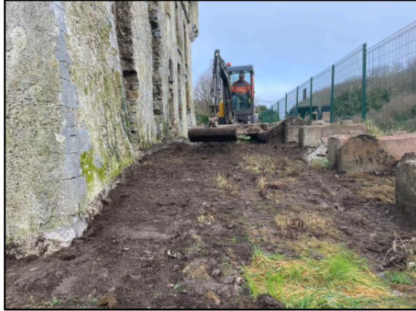
Plate 20: Exterior of building from S after removing architectural fragments and backfilling.
