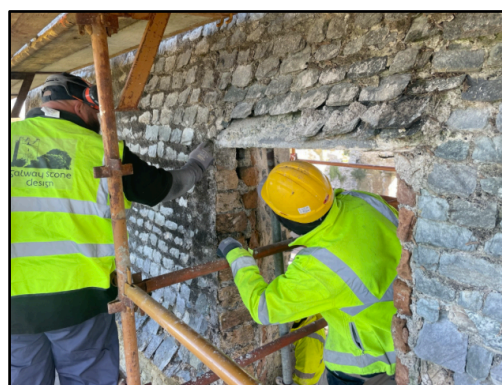
Plates 8 & 9: Repointing of joist hole and work on external finish on upper levels of building.
