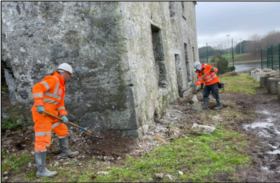
Plate 4: Removing debris after scaffolding removed. Taken from NW.
