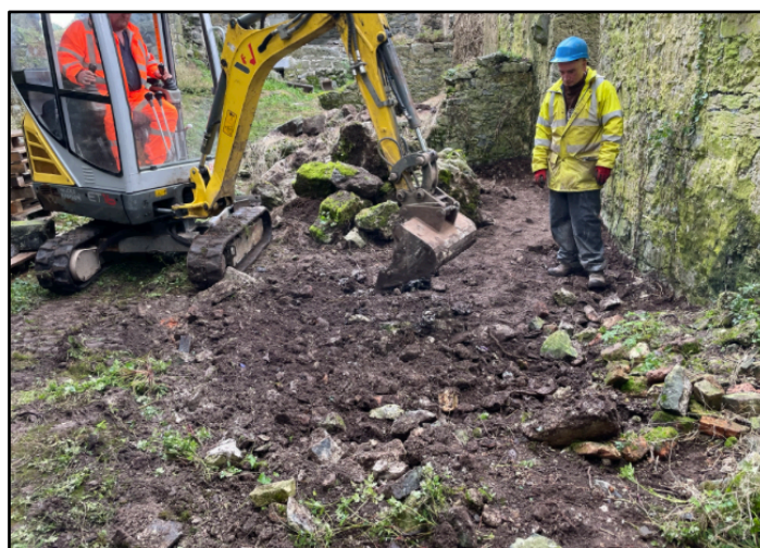
Plate 13: leveling of rubble in SE of site.
