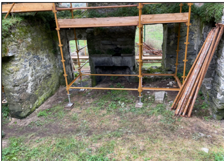
Plate 3: Scaffolding being erected on interior of W wall of building.
