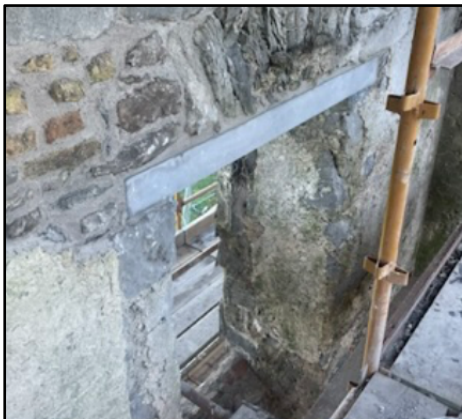
Plates 5 & 6: Lintels replaced and repointing above window openings.
