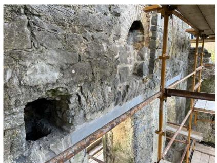
unsuitable bedding to ensure good adhesion. Sound slates were left in place. Works will proceed so as not to disturb nesting birds or their nests. During this phase, suitable stone was retrieved from piles in the east range under archaeological supervision where it fell following the fire in 1910, for use in the consolidation of the openings and pinnacles. Unfortunately, very little stone cappings for the pinnacles were identified, perhaps having been taken off site following the fire.
